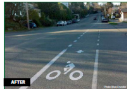
Nickerson Street - Seattle, WA road improvements
